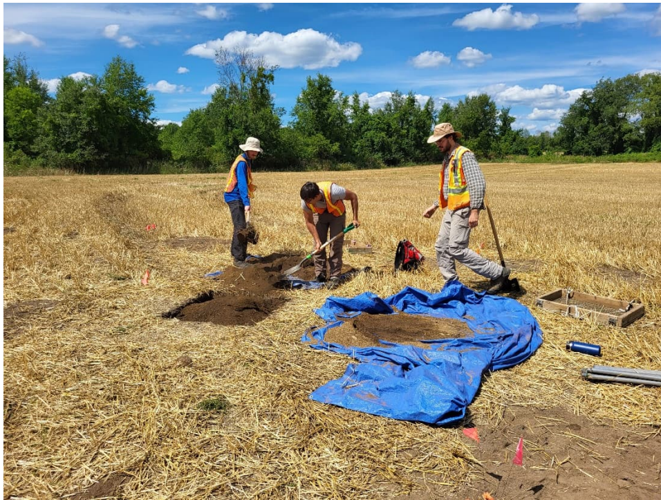
Image 3: Site backfilling in progress; facing northwest, August 15, 2022
